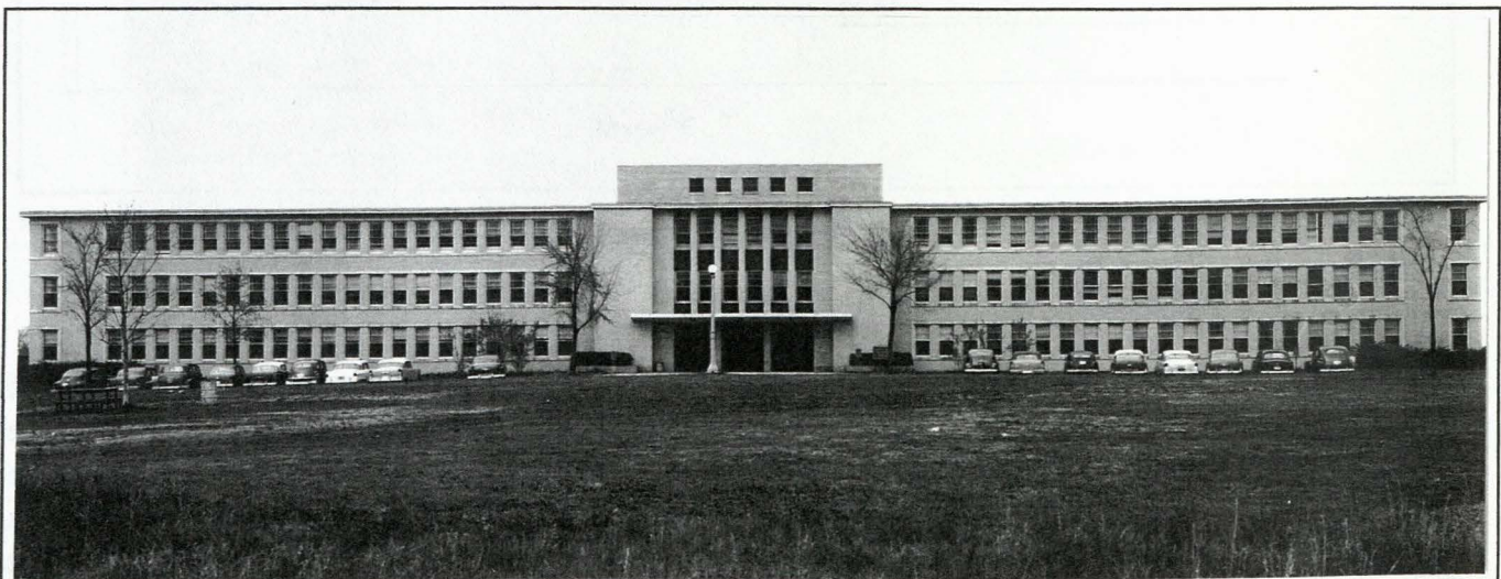
Figure 12. Federal Office Building No. 4 in Suitland, Maryland. Picture taken facing east.
